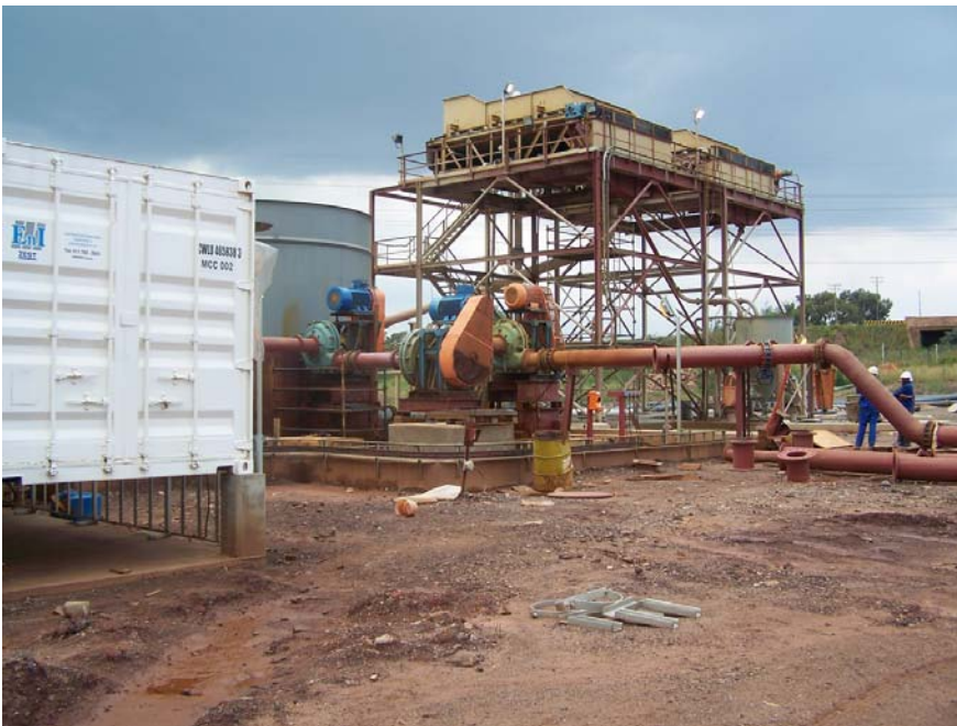
Large pumps bring water to the dump site to create slurry.
