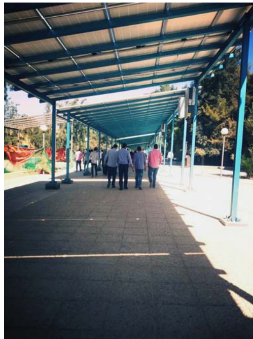
A 616 kW canopy system throughout the campus also provides welcome shade for pedestrians.
